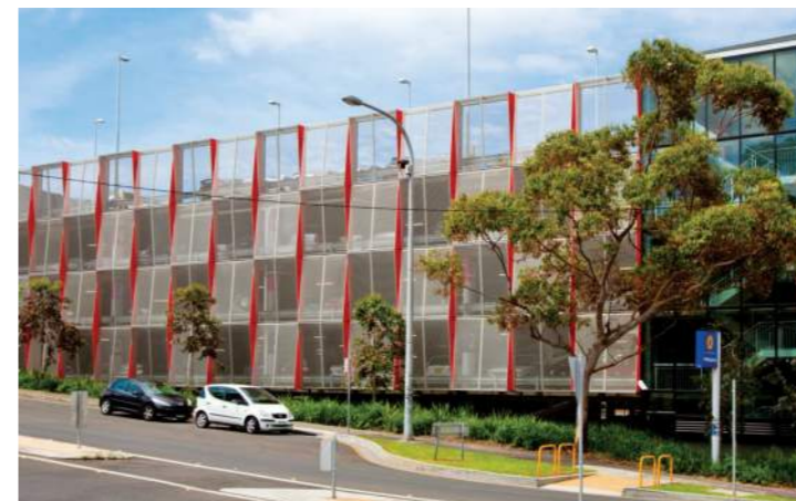
WOLLONGONG RAILWAY STATION CAR PARK Sydney, NSW, Australia
