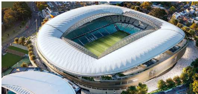
ALLIANZ STADIUM Sydney, NSW, Australia
